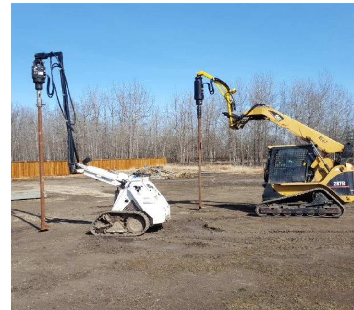
Installation of a helical pile today
